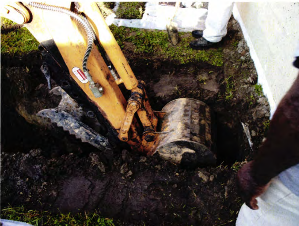
Picture 2: UST 466Dogwood excavation in progress .
